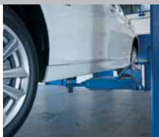
POWER LIFT HL 2.30 NT DT – short lifting arm with 2-times telescopic arms provide more adjustable range and simplifies lifting of shorter and wider vehicles
