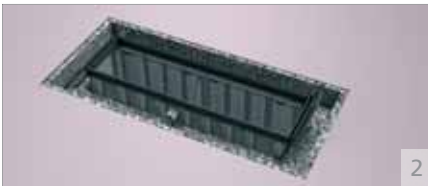
Picture 2: Uncover the concrete around the installation canister
