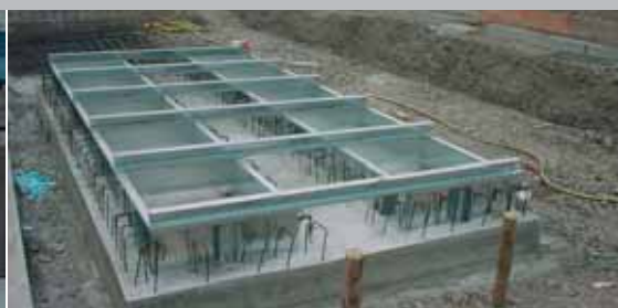
Example picture: installation cassette Optional with park position for axle jack
